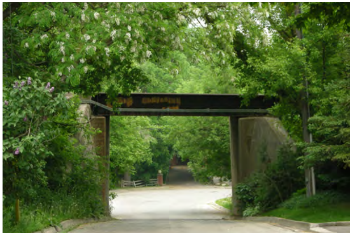
William Street - Rail Bridge
