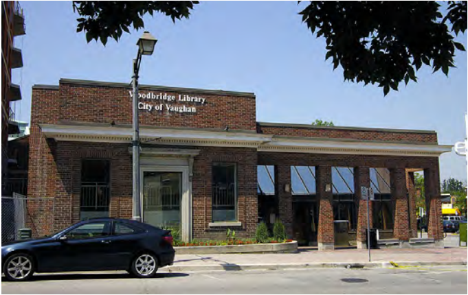
Heritage Building - Woodbridge Avenue
