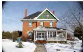
8127 Kipling Avenue Listed in LSHS + Note #'s 8066, 8074 + 2.5 Storey, Built as Manse + Queen Anne/Edwardian, 1902 + Romanesque detailing + Stone Arches + Bracketed Cornice + Portico and Wrapping Verandah + Shingled Gable
