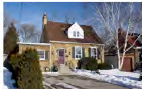
8227 Kipling Avenue + 1.5 Storey + Victory Housing, Circa 1950 + Buff Brick + Single Central Dormer + Later Garage Addition
