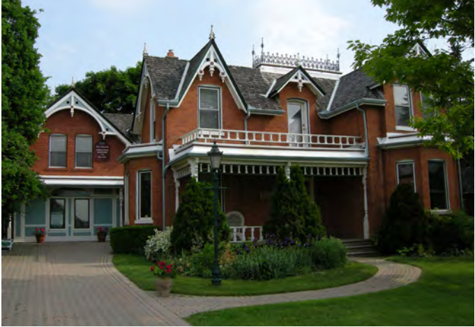
Heritage Building - Woodbridge Avenue
