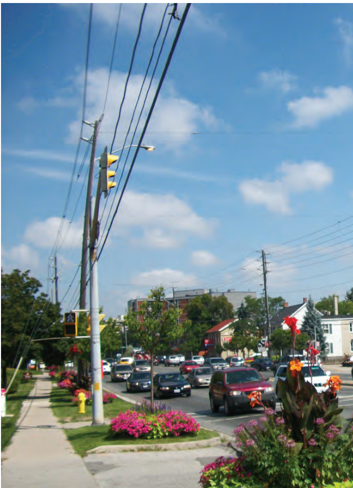
Street with Overhead Hydro Wires
