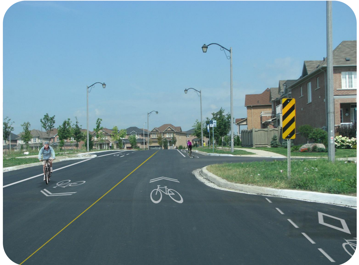
Combination of Sharrow and Bike Lane Pavement Markings
