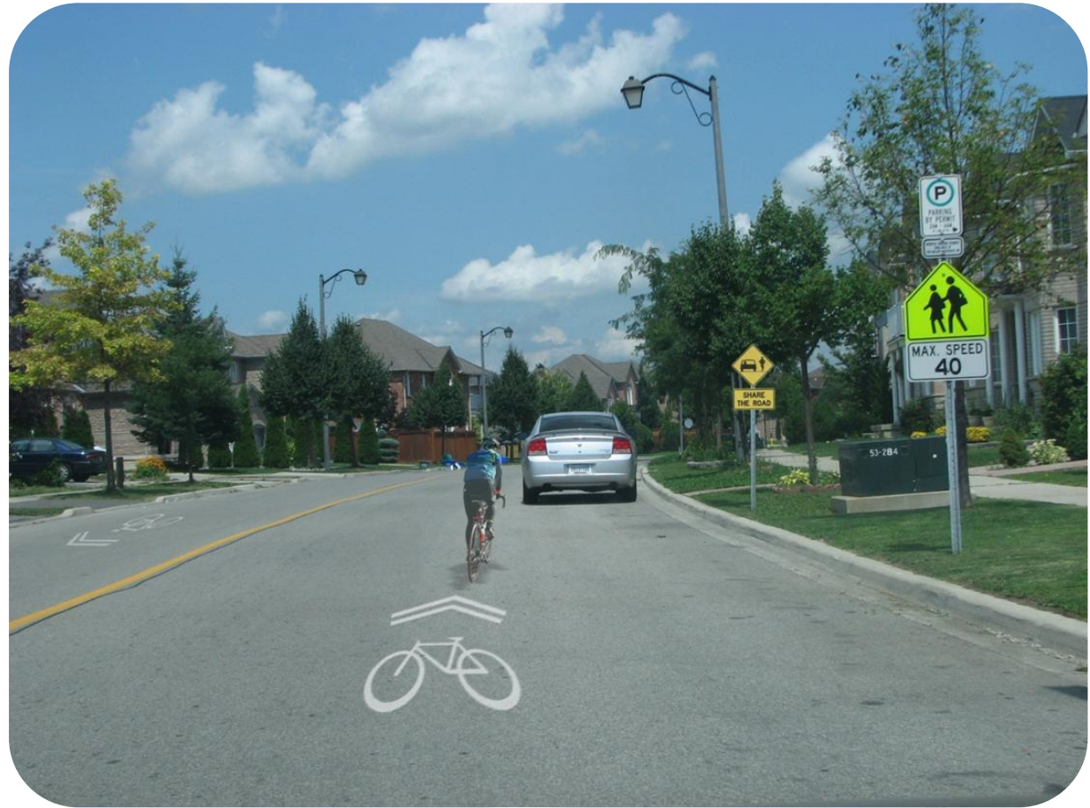
Sharrow Pavement Markings
