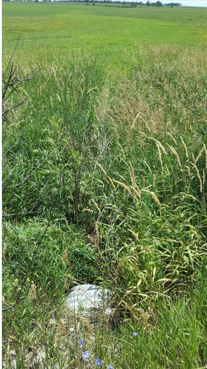
Photograph 4 – View of West Don River culvert looking South near Borehole 20-03
