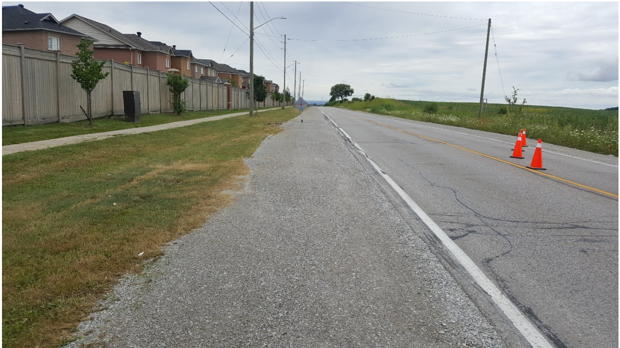
Photograph 10 – Kirby Road looking west from Borehole 20-09
