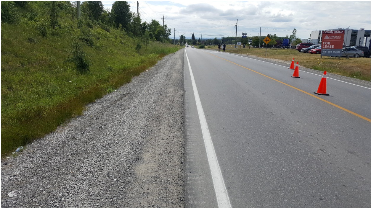
Photograph 8 – Kirby Road looking west from Borehole 20-07
