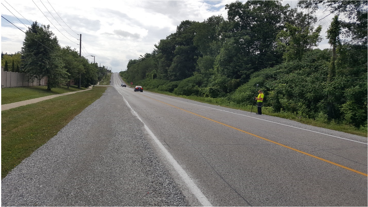
Photograph 13 – Kirby Road looking west from Borehole 20-11
