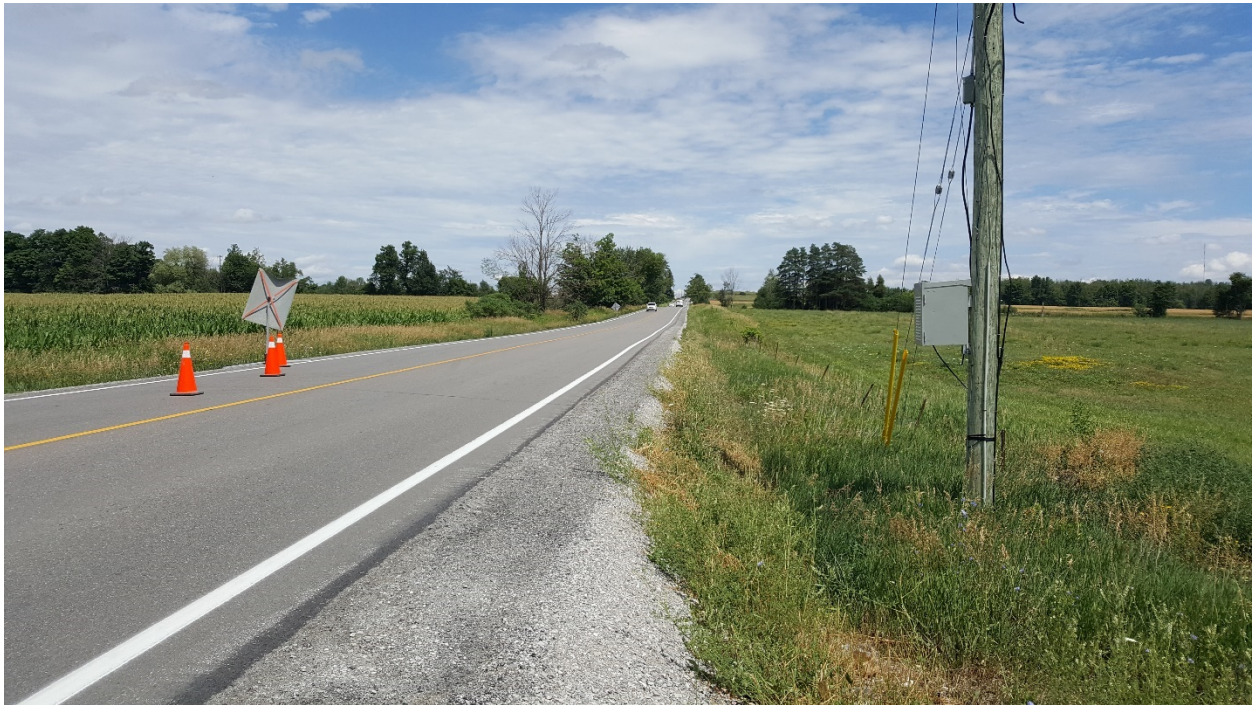
Photograph 2 – Kirby Road looking east from Borehole 20-03
