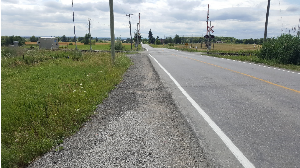
Photograph 5 – Kirby Road looking west at Go Rail line near Borehole 20-06
