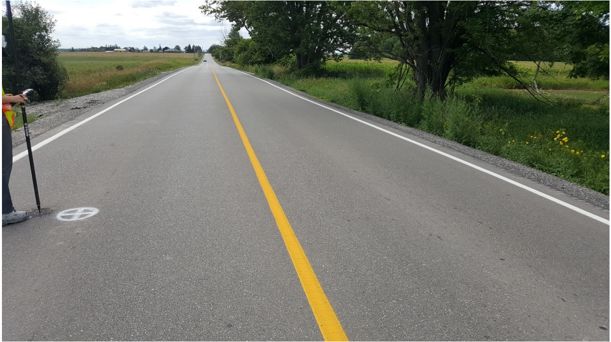
Photograph 3 – Kirby Road looking west from Borehole 20-03
