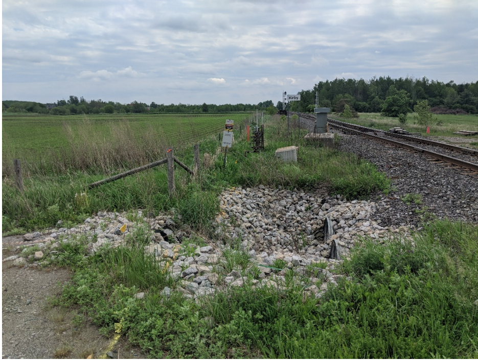
Photograph 7 – Barrie Go Rail line crossing Kirby Road looking south
