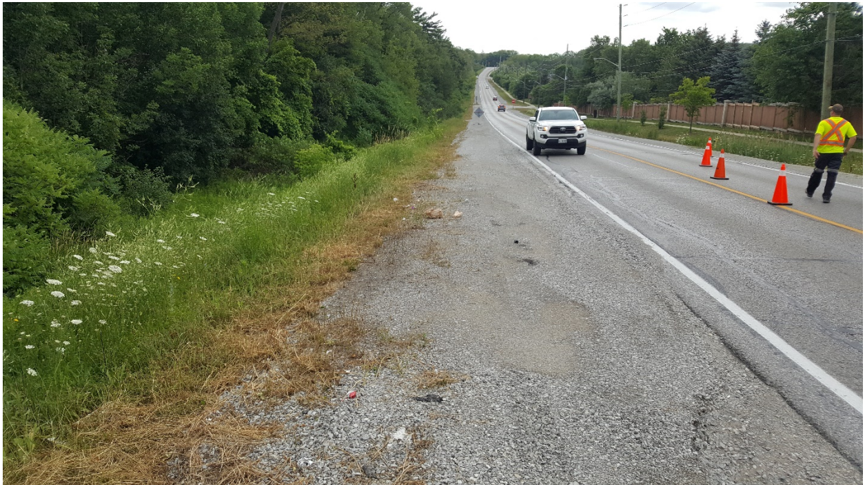
Photograph 12 – Kirby Road looking east from Borehole 20-10
