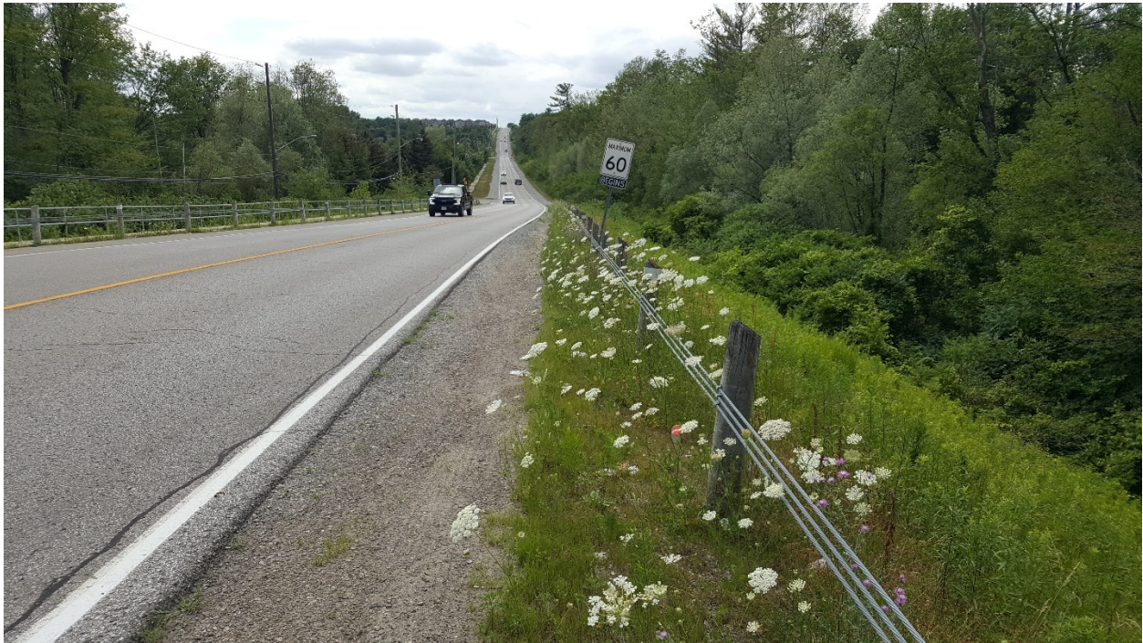
Photograph 14 – Kirby Road looking west from Borehole 20-12
