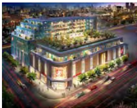
A Proposed Home Depot at Queen St W and Portland St, Toronto
