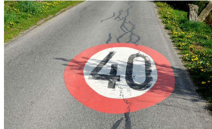
40 Km/H Pavement Marking
