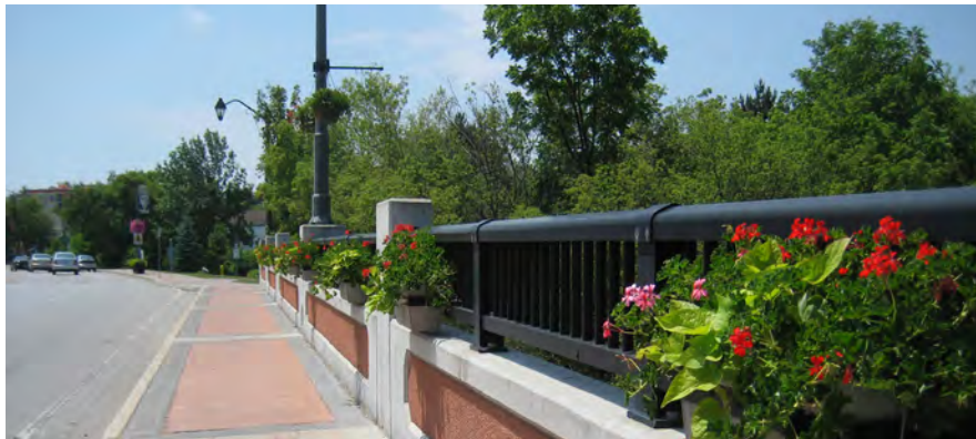
Bridge over the Humber River in Woodbridge
