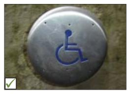
Large circular power door operator control, clearly marked with International Symbol of Accessibility.
