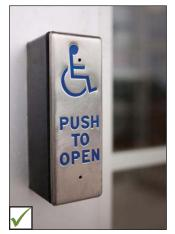
Example of rectangular shaped power door operator control used in retrofit situations only.
