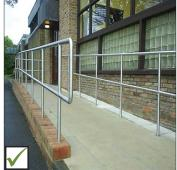
Ensure handrail extensions do not obstruct path of travel or create hazards.
