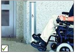
Long extended power door operator control can accommodate a wider range of users (e.g., can be operated by foot or foot rest).
