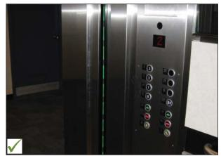
*Elevator sensor door and floor registration buttons.*
