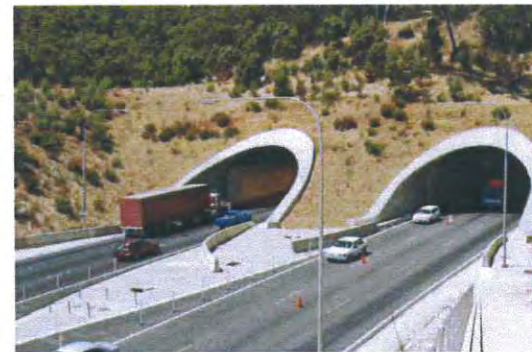
Twin Bored Tunnel
