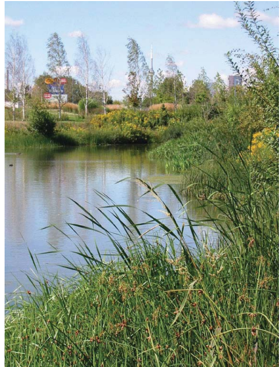
Stormwater ponds appropriately integrated with adjacent industrial land uses and enhanced through naturalized planting.
