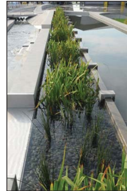
Bioswale Sherbourne Common Toronto, Canada
