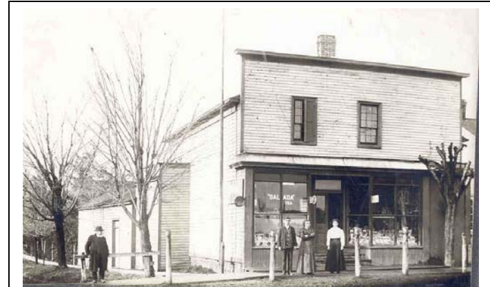
The Bailey Store. A false front on a gabled village shop mimics the form of a town shop. Photo from the Vaughan Archives.
