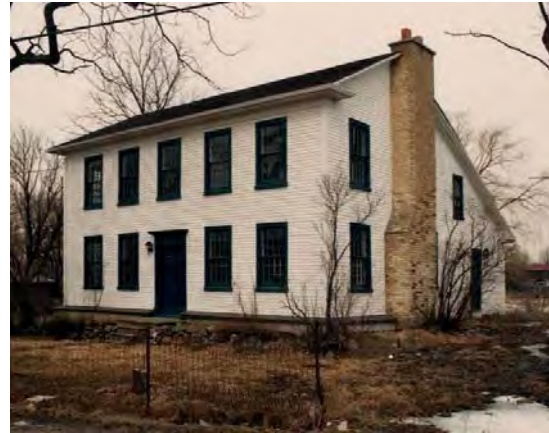
The 1815 Fulton-Vanderburgh House in Richmond Hill, after restoration.
