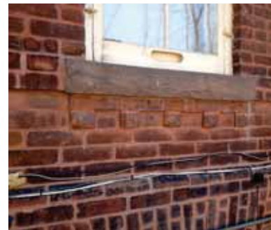
27. Window sill and corbelled brick detail, north elevation (ERA)
