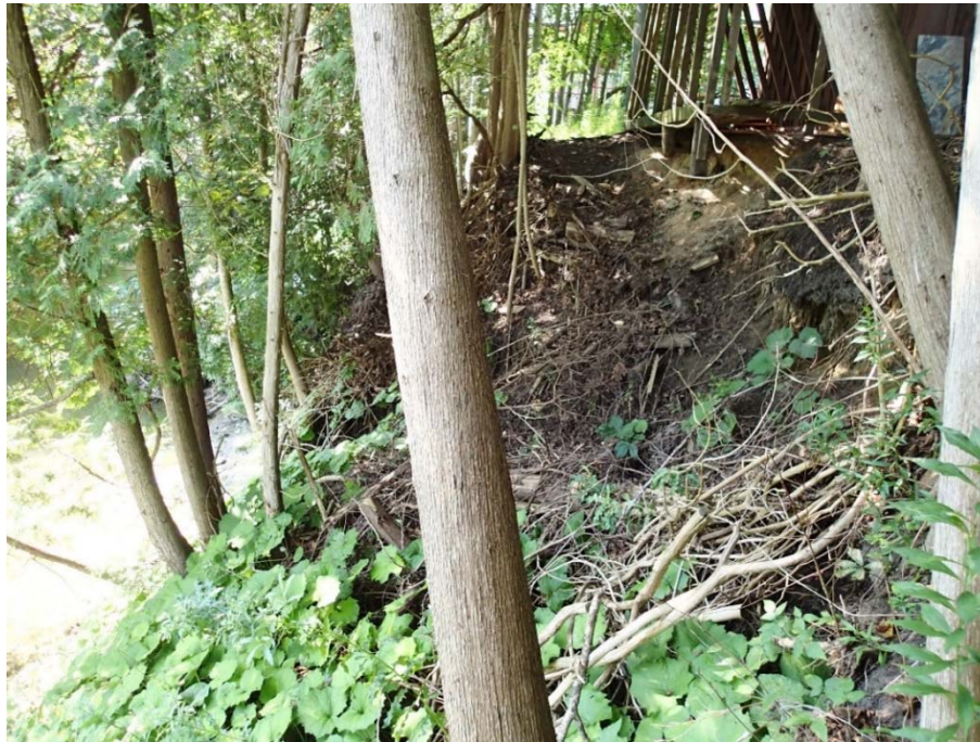
Photo 1. Active slumping along west bank below outbuilding at 75 Valley Road
