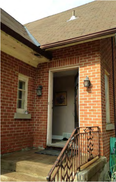
'Photo E-3', Spalling Bricks at Entry Porch
