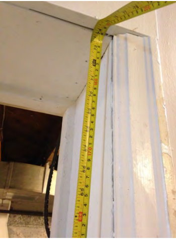
'Photo B-3', Height of Door Openings
