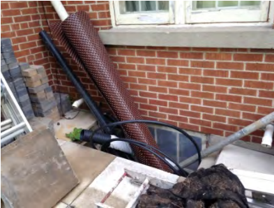
'Photo E-8', Blocked Window Lightwell
