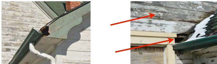
Above: Deterioration of the wood cladding and fascia board on the south elevation
