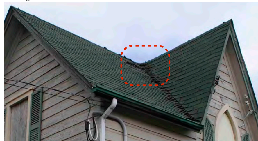
Above: Porch exhibits substantial damage to asphalt shingles which may also be responsible for wood deterioration below this surface. An invasive exploration will be required to determine the extend. Below: Roof shows further damage of shingle covering.
