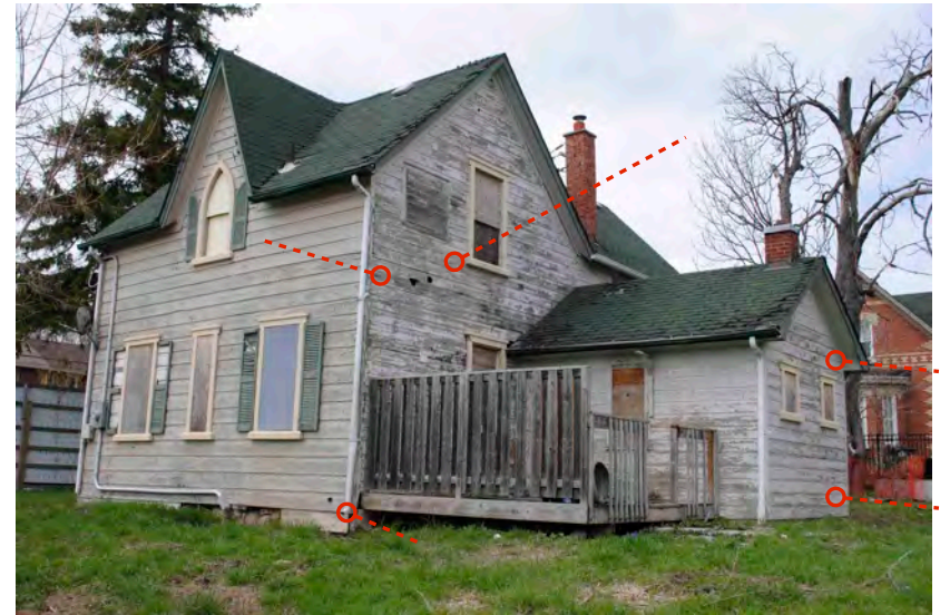
Above and Below: South and east facade exhibits wood cladding condition with areas of deterioration and openings. It is evident that different degrees of deterioration have occurred in wood elements of the building.
