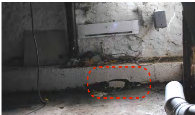
Above: Deterioration of concrete foundation on the east elevation.
