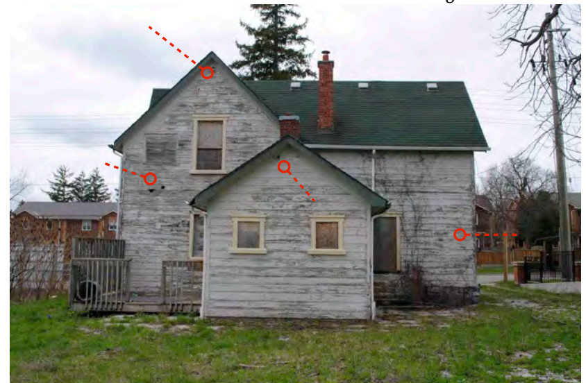
Above and Below: South and east facade exhibits wood cladding condition with areas of deterioration and openings. It is evident that different degrees of deterioration have occurred in wood elements of the building.
