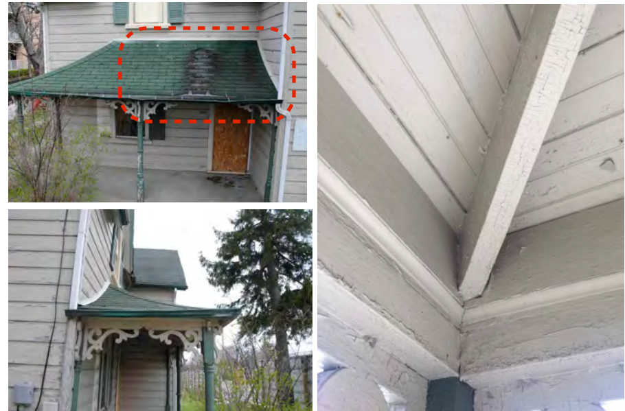
Above: Porch exhibits substantial damage to asphalt shingles which may also be responsible for wood deterioration below this surface. An invasive exploration will be required to determine the extend. Below: Roof shows further damage of shingle covering.
