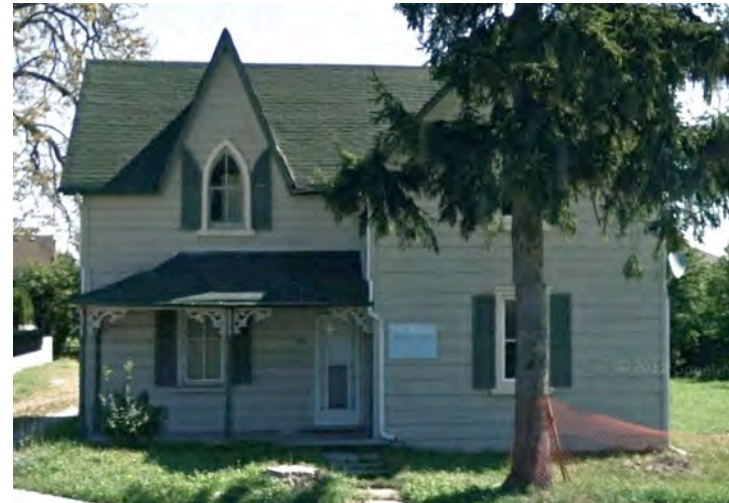
Above: Front (West) facade showing asymmetrical composition with pointed gable and lancet window over the wooden porch. 2013
