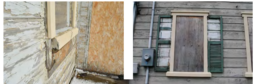
Above left: Deterioration of the styrofoam surrounds and peeling paint on the south elevation
