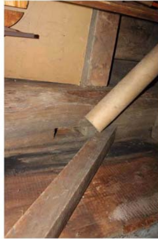
South-West corner post at south bracing detail. Nailed connection and mortise no longer in use.
