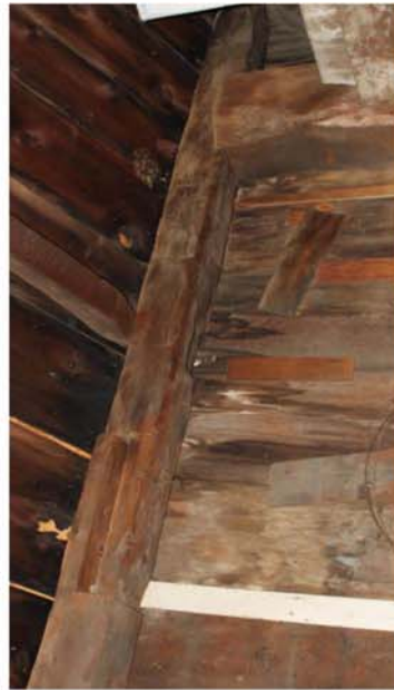
West wall. Note pinned lap joint on top plate, notched connection at post and tapered rafter at top plate.
