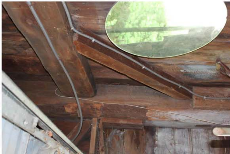
South-East corner post, bracing and girder connection. Note mortise and tenon and pin.
