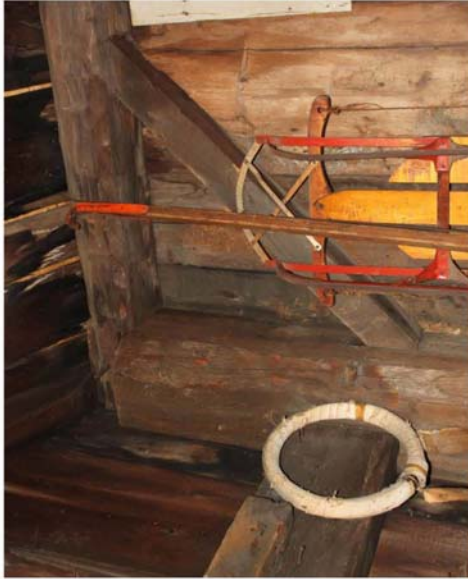
South-West corner post at west bracing detail view. Mortise and tenon joinery. Note post and girder connection with pins.
