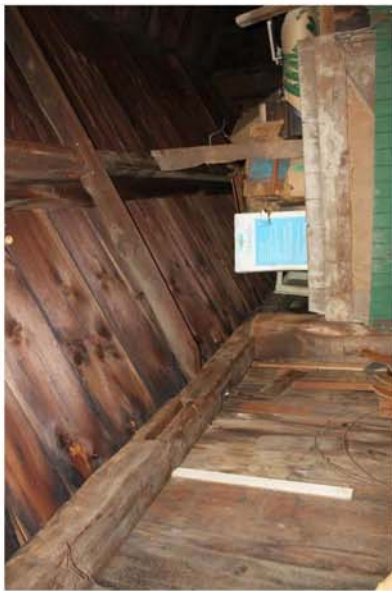
Detail of reinforced mortise and tenon joint at rafter with purlin. Note nails.
