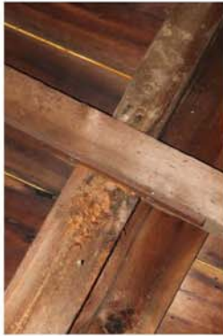
Detail of reinforced mortise and tenon joint at rafter with purlin. Note nails.
