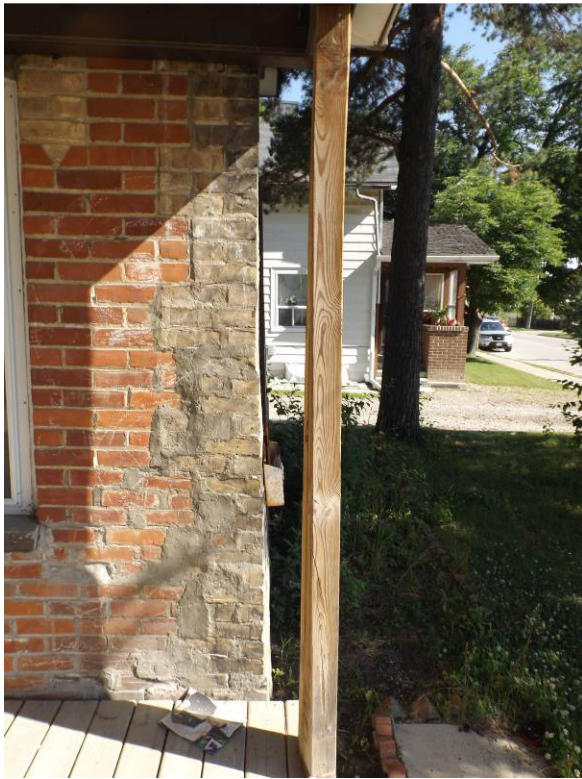
Figure 10. Desperate repairs to masonry at the northeast corner.
