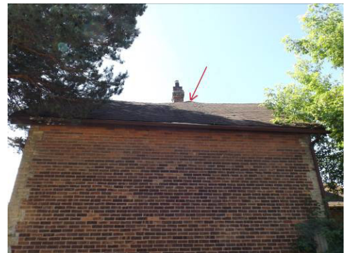
Figure 8. The north wall of the original house is windowless. The bump in the roof ridge due to the raising of the cross ridge is visible just to the right of the chimney.
