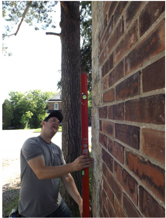
Figure 12. Northeast corner out of plumb in north-south direction.
