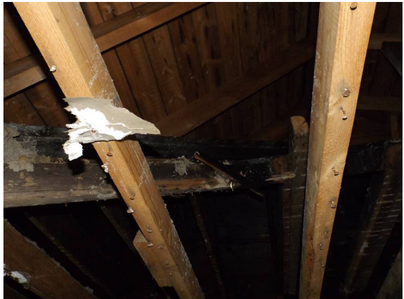
Figure 17. Evidence of a fire: Extensive charring over the back bedroom in the second floor.
