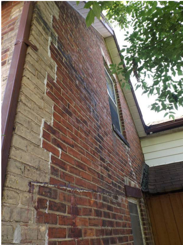
Figure 11. Northwest corner. Note also stepped crack between the windows.
