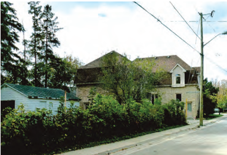
PHOTOGRAPHS (A-C) OF SUBJECT PROPERTY AND SURROUNDING AREA
