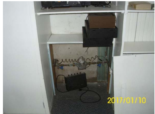
Entering water main and meter at south- east corner of Basement
