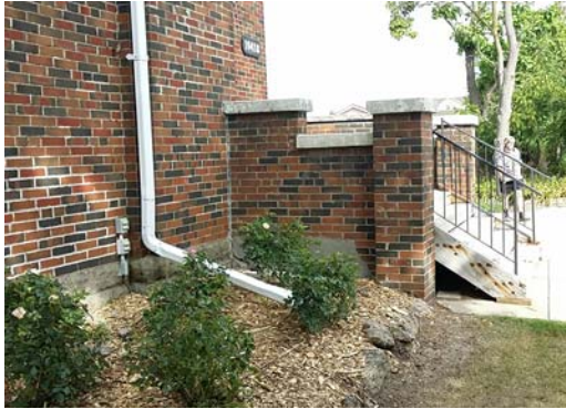
Northeast stair – temporary wood stair bearing on sidewalk
