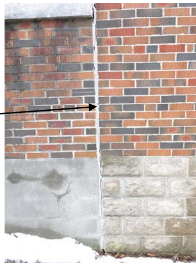
Exterior East Stair- Gap at Church wall
