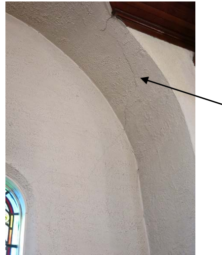
Cracks at transept arches
