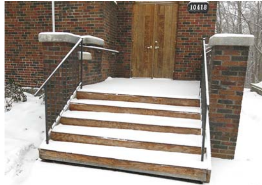
Temporary wood stair between existing masonry side walls.
