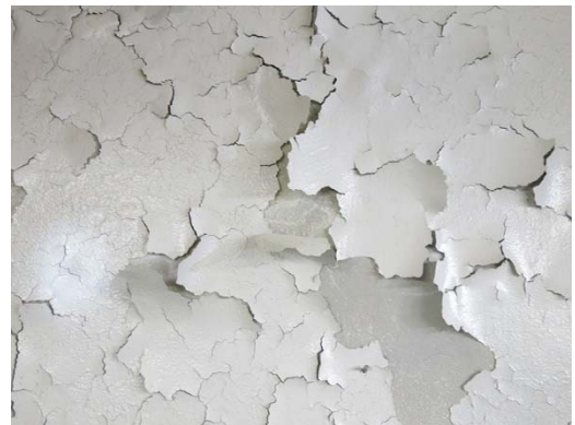
Peeling paint in Basement
