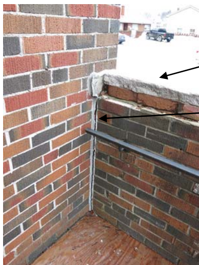
Exterior East Stair- broken coping & Gap
