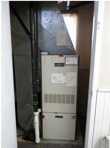
Existing forced air gas fired furnace
