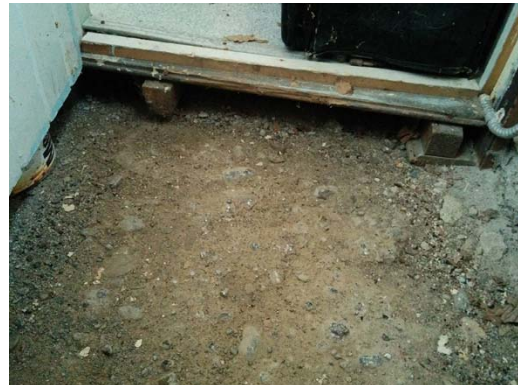
Space below existing NW stair at door to kitchen shows existing 2x2 sleepers at 16" o.c. with wood floor above.
