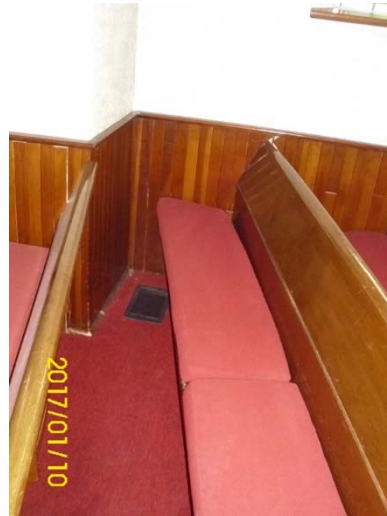
Typical floor register serving main floor throughout perimeter
