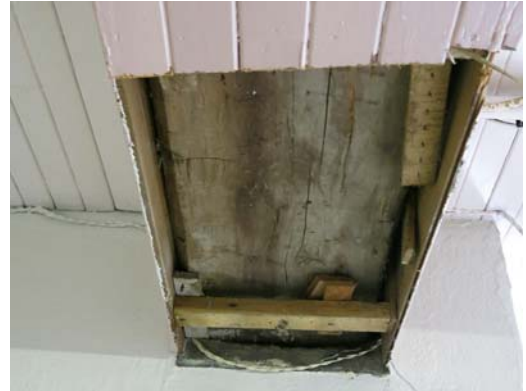
Underside of wood beam exposed
