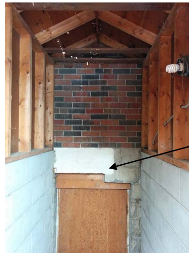
South concrete stair door to church with cantilevered lintel
