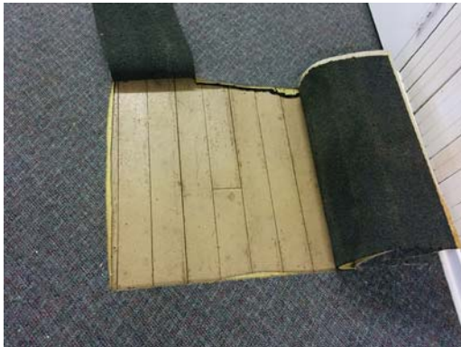
Test hole in existing carpet at Basement level wood floor below
