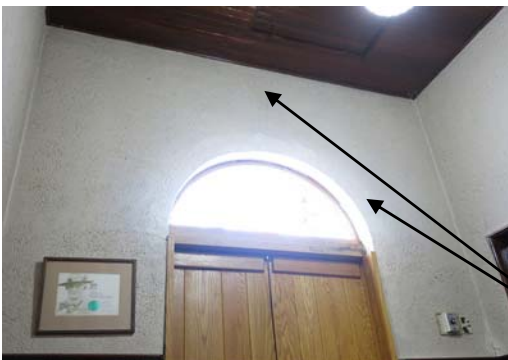
Cracks in plaster above East Entry Arch
