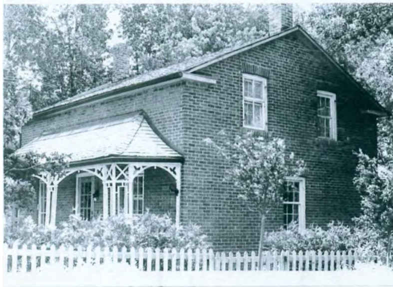
Figure 2. North façade, 1970s Original 6/6 windows still in place, with a 2/2 storm on the upper left window.
