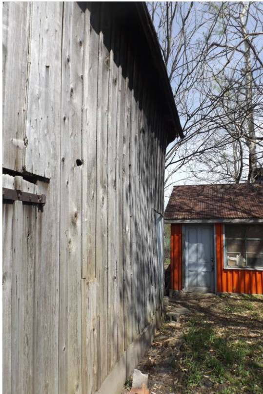
Figure 16. East side of barn showing bowed wall. Steel shed to the rear.
