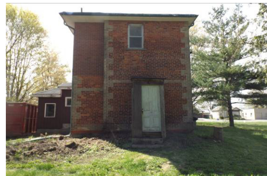
Figure 11. View from the north. Ad-hoc frame rear vestibule. Original brick on the right, and at ground floor on the left. Window opening not original.
