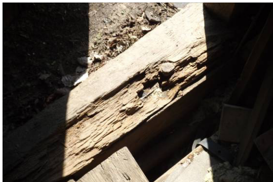
Figure 17. Rot in the timber sill of the barn.
