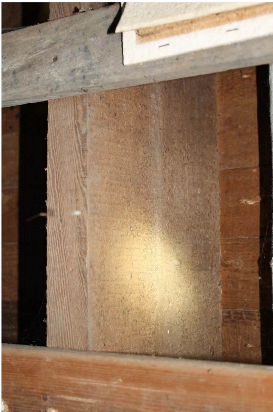
Ground floor joist with vertical saw marks
