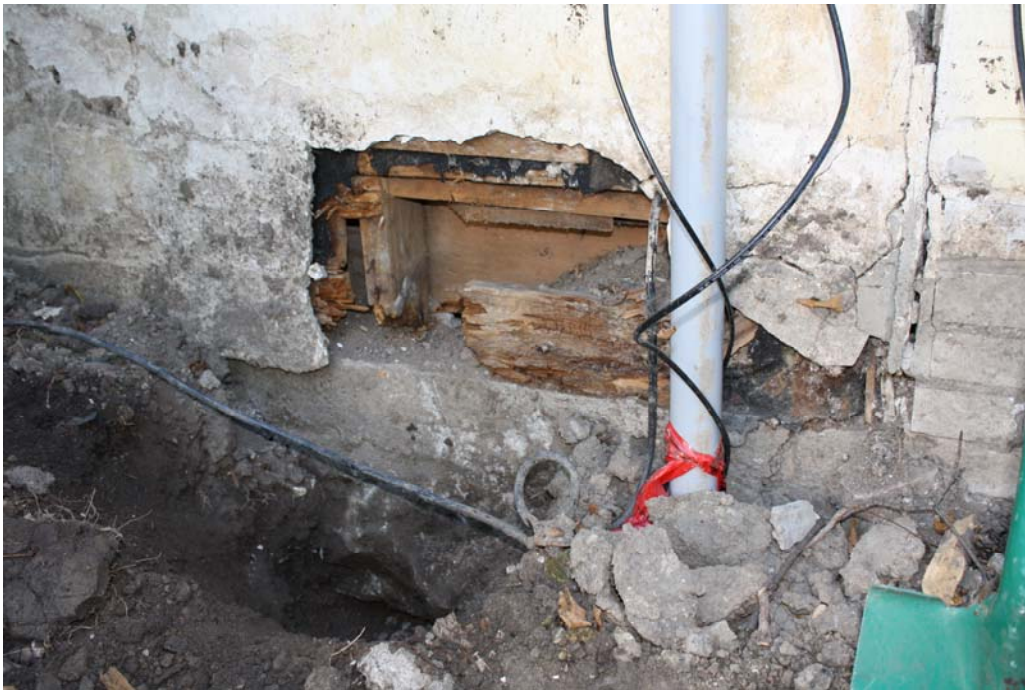
West elevation: foundation at framing condition.
