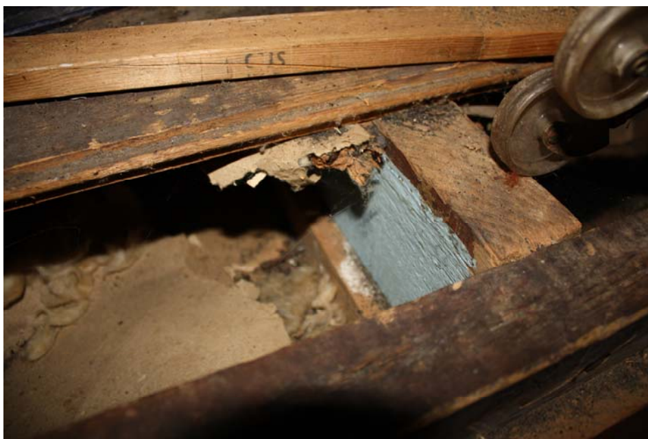
North section attic, tongue and groove floor boards.
