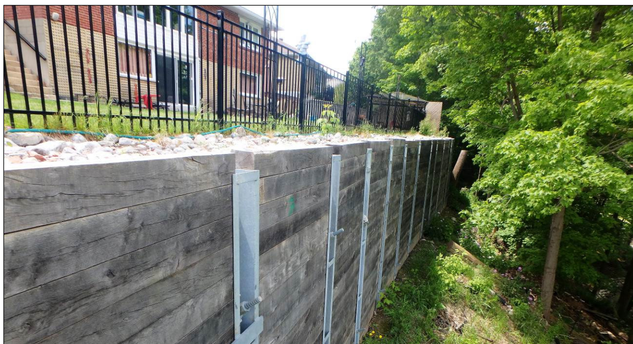
Figure 3. Soldier pile with timber lagging wall to protect houses in Toronto managed by TRCA. Source: TRCA, 2017.
