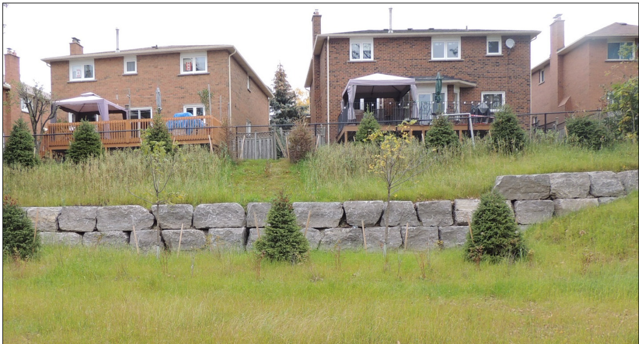
Figure 2. A gravity retaining wall to protect houses in Vaughan managed by TRCA. Source: TRCA, 2017.
