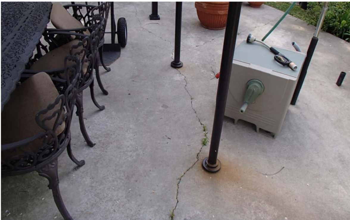
Cracking in concrete pad
