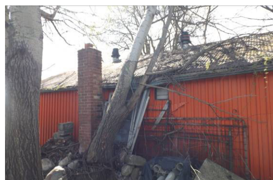
Figure 20. Tree fallen against north wall and roof of the steel shed.
