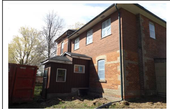
Figure 9. View from northeast. Window at lower right is the only original opening in the tail. The frame entry porch is recent.
