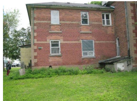
Figure 10. View from west. Original brick, but no original window openings.
