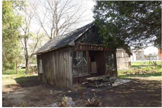
Figure 12. Front (south) side of the small outbuilding. Large 6-pane windows flank a recessed glazed entry door. Sagging wall and roof are evident.
