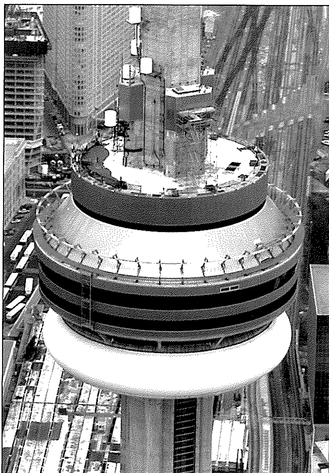
Scaffolding installation at the top of the CN Tower. Photo provided by Skyway Canada Scaffolding.
