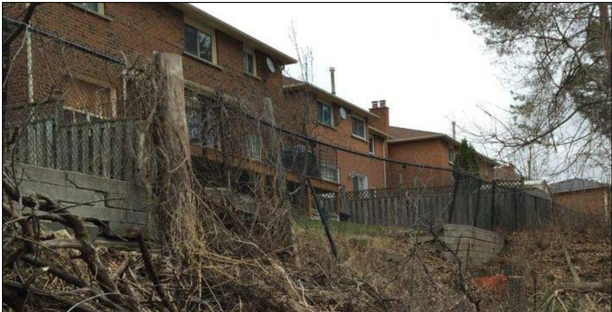
Figure 1. Slope movement and failed concrete retaining wall near 28 Jason Street. Source: City of Vaughan, unknown date.
