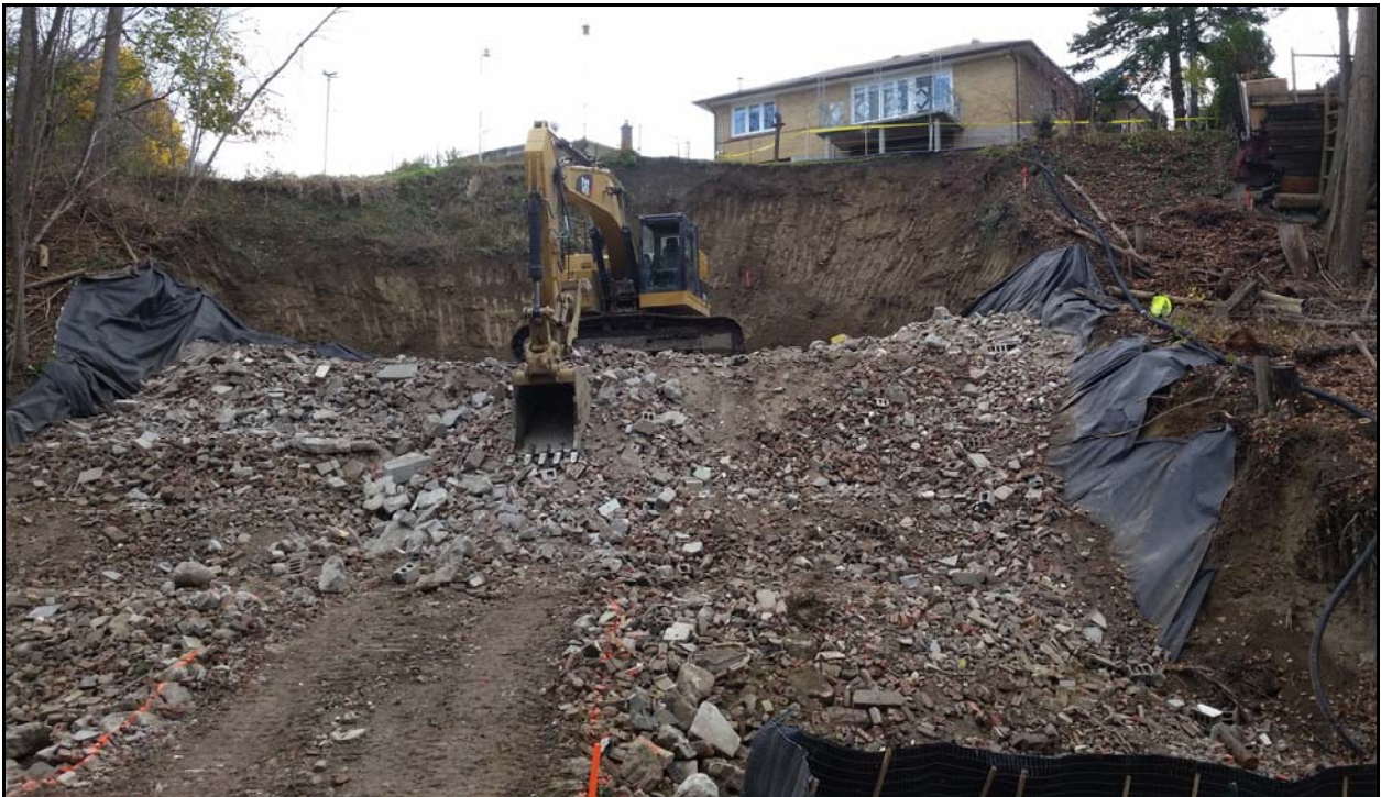
Figure 3. Clean fill being used to in-fill the erosion scar. Source: TRCA, 2014.
