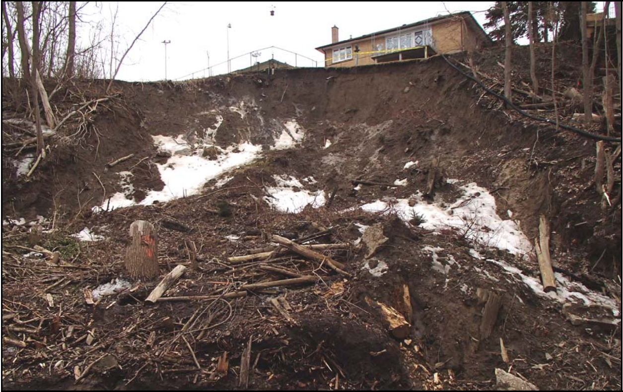
Figure 2. A TRCA project site experiencing erosion and slope instability. Source: TRCA, 2014.
