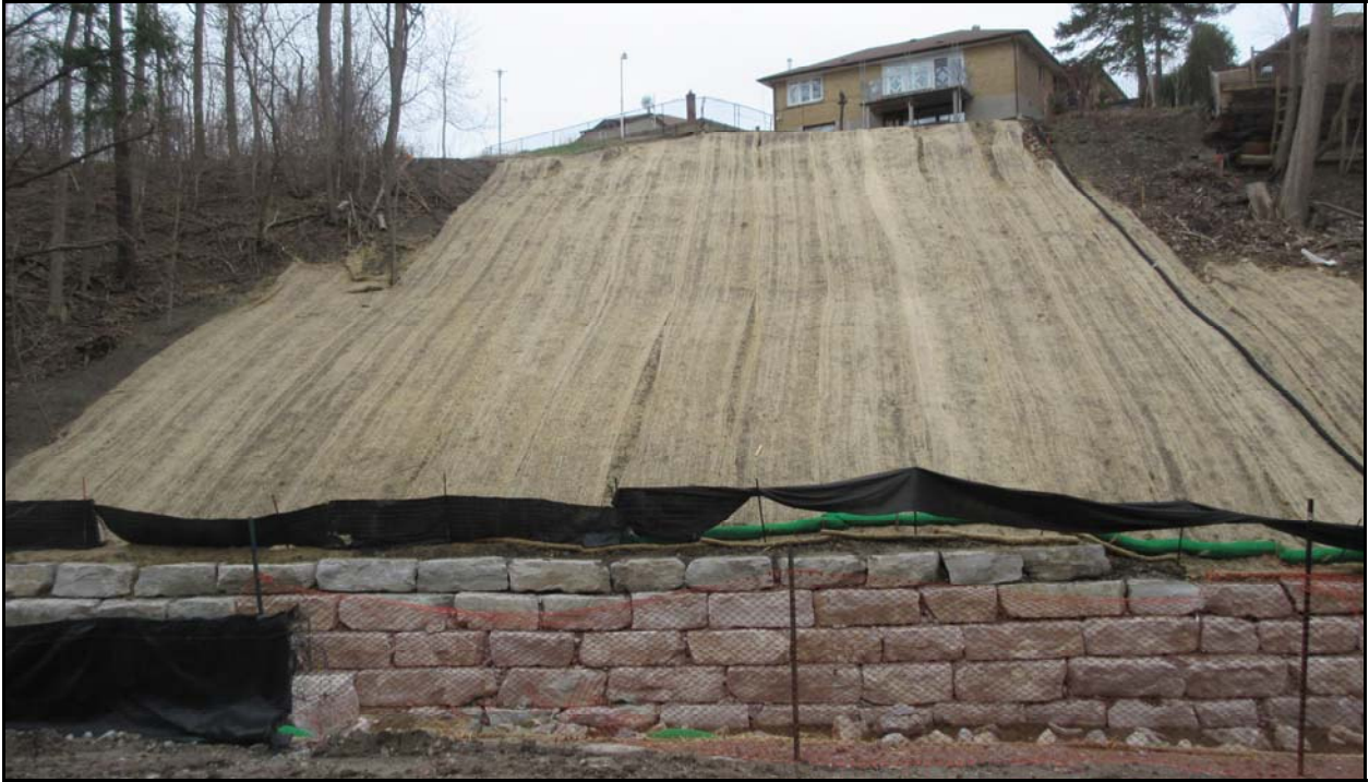
Figure 4. Stabilizing the slope with erosion matting prior to planting. Source: TRCA, 2015.
