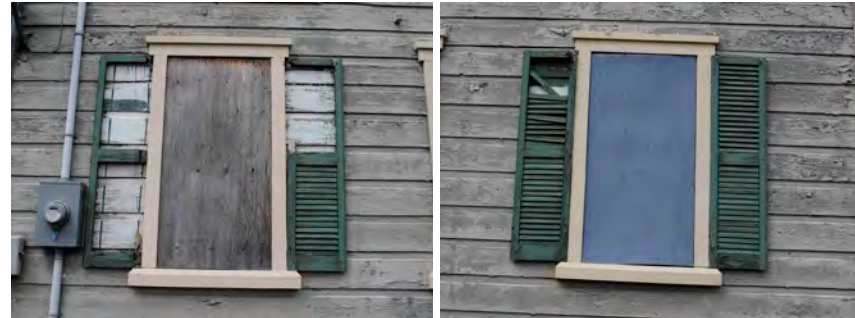
Above and Below: Rapidly deteriorating condition of shutters on east facade, compared with relatively good condition of shutters on the west facade below.
