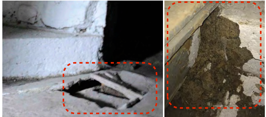
Above: Location of significant deterioration/buckling of the concrete floor before entry to boiler room, to the left. At the right, concrete foundation deterioration at foot of stair.
