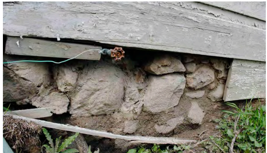
Below: Significant deterioration of mortar joints of rubble foundation on the north facade.
