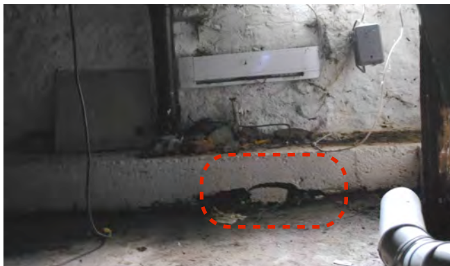
Above: Deterioration of concrete foundation on the east elevation.
