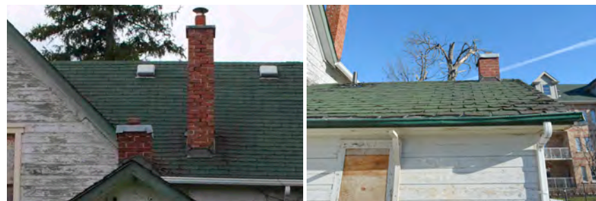
Above left: Some water staining is visible on the roof. The mortar joint on the chimney are severely deteriorated.
