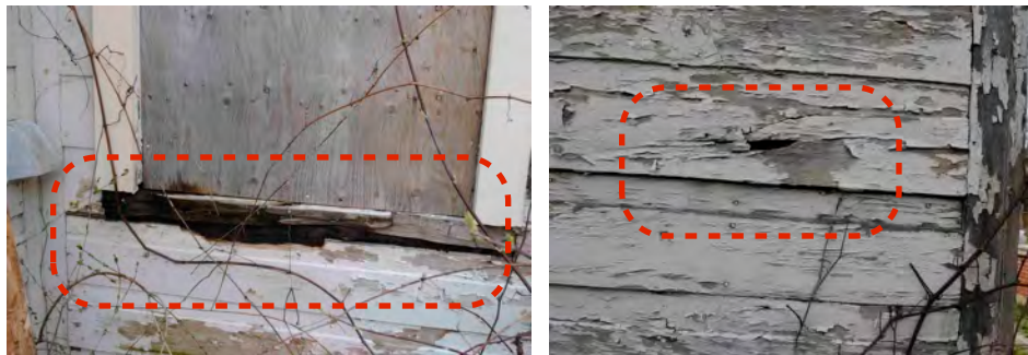
Above: Detail of wood cladding deterioration, peeling paint, and sill rot noted on the east elevation.
