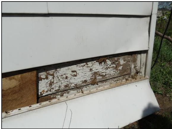
Figure 9: Exposed wood clapboard beneath metal cladding, 2016
