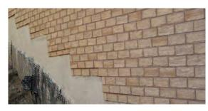
Veneer Should Be Stepped to Follow Sloping Grade to Limit Exposure of the Foundation Wall (image shown prior to backfilling with topsoil)
