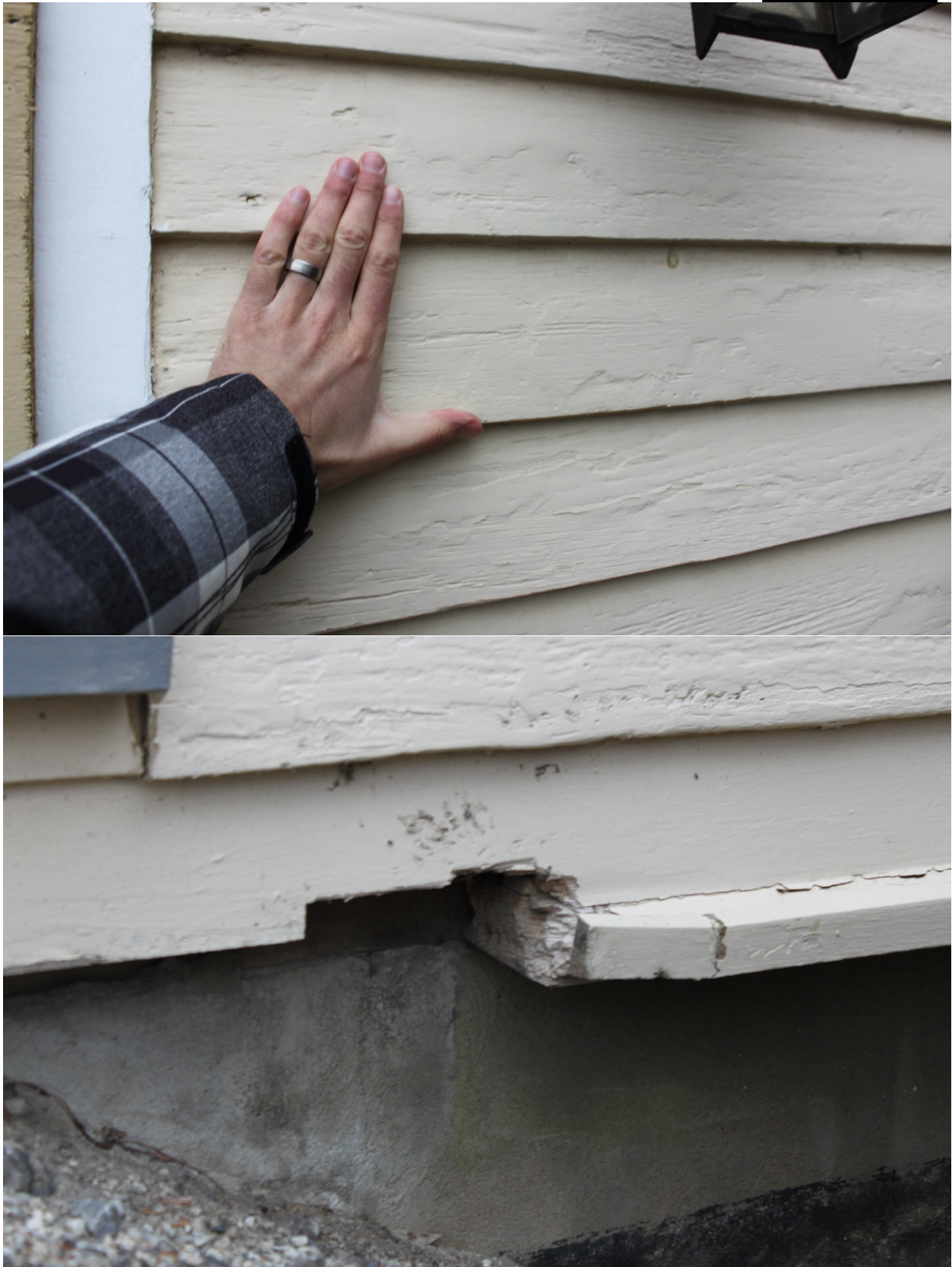
Details of 4inch clapboard panels and poured concrete foundation from 1980s. December 23, 2014
