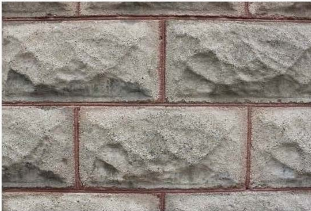
Bottom: 229 Pine Grove Road close up of blocks. The pattern matches exactly that of the Sears machine. Note red tinted mortar joints troweled with bead.
