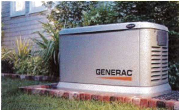
Gas-fired Generators
