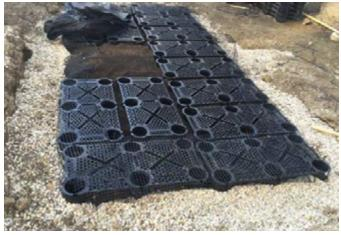
Use of a soil cell system provides extra support for greater compaction of hard surfacing of sidewalks, to protect the soil medium for healthy tree growth.
