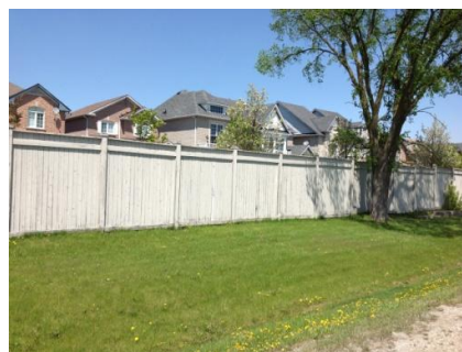
Board on board fence along north edge of the Precinct
