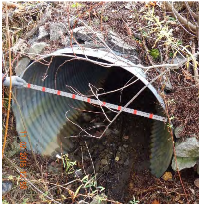
1200 mm CSP culvert between Reaches EPC-2 and 3.
