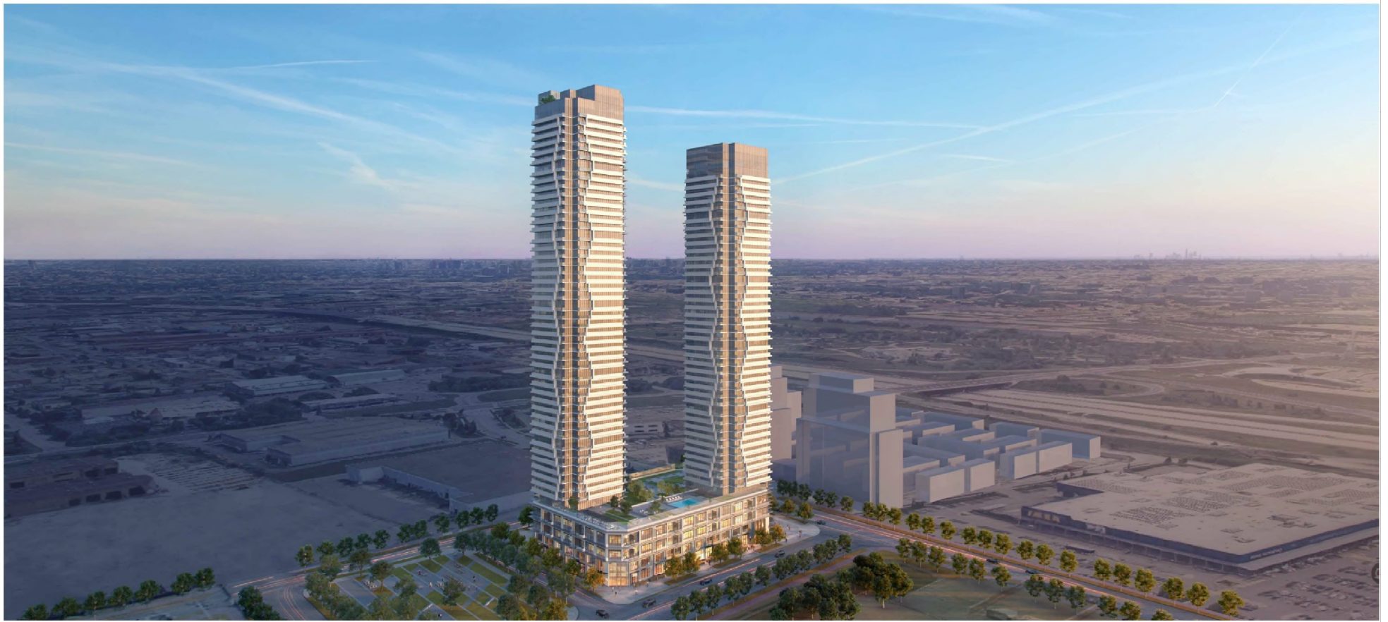
View Looking South-East
