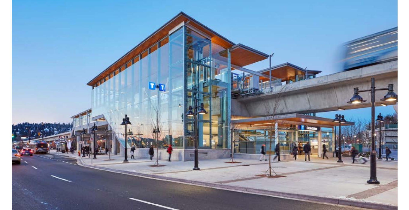
Evergreen Line Station, Coquitlam, Canada
