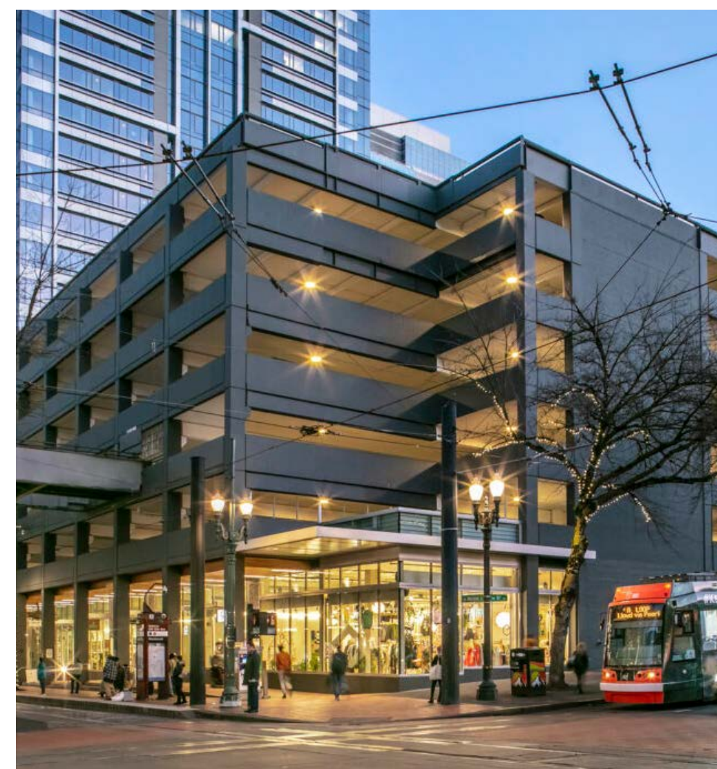
Yamhill Parking Garage and Retail, Portland
