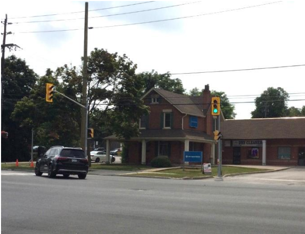
Photo 17 Edwardian influenced residence, 7666 Yonge Street, looking southwest
