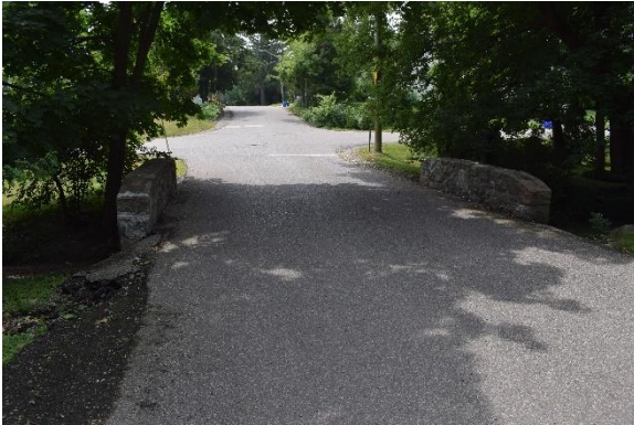
Photo 31 Bridge over creek on Elizabeth Street, looking south
