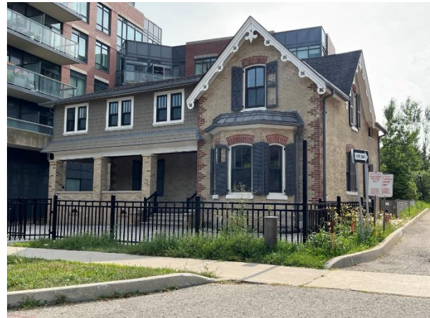
Photo 12 Structure with medium heritage integrity, 7616 Yonge Street, looking west
