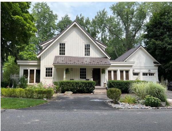
Photo 13 Structure with low heritage integrity, 143 Brooke Street, looking north
