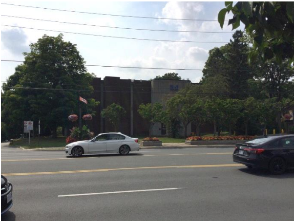
Photo 23 Brutalist structure, 7700 Yonge Street, looking west
