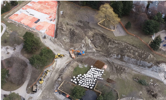
Underground SWM facility under construction Gallanough Park, Vaughan
