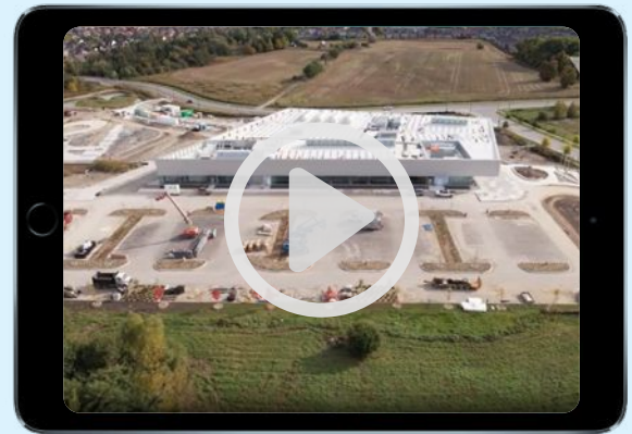
Construction update: Carrville Community Centre
