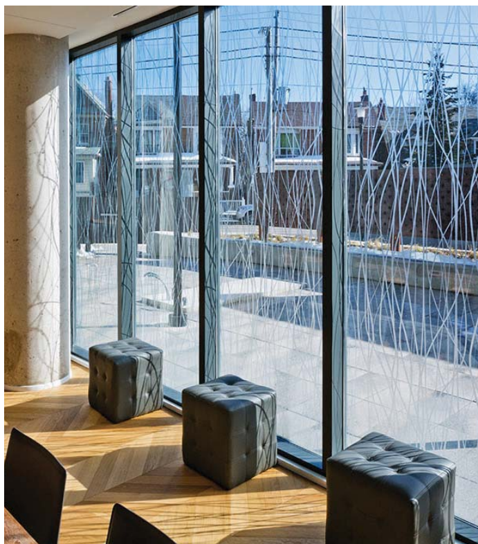
Treated glass to prevent bird strikes. (Image Credit: 60 Howard Park Ave, Toronto, RAW Design. Photo courtesy of Walker Textures)
