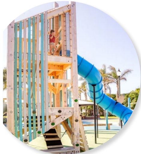
1 THE TIMBER TOWER FOR COMBINED PLAY – INCLUDES CLIMBING WALLS, POLES, ROPE, AND TALL SLIDE
