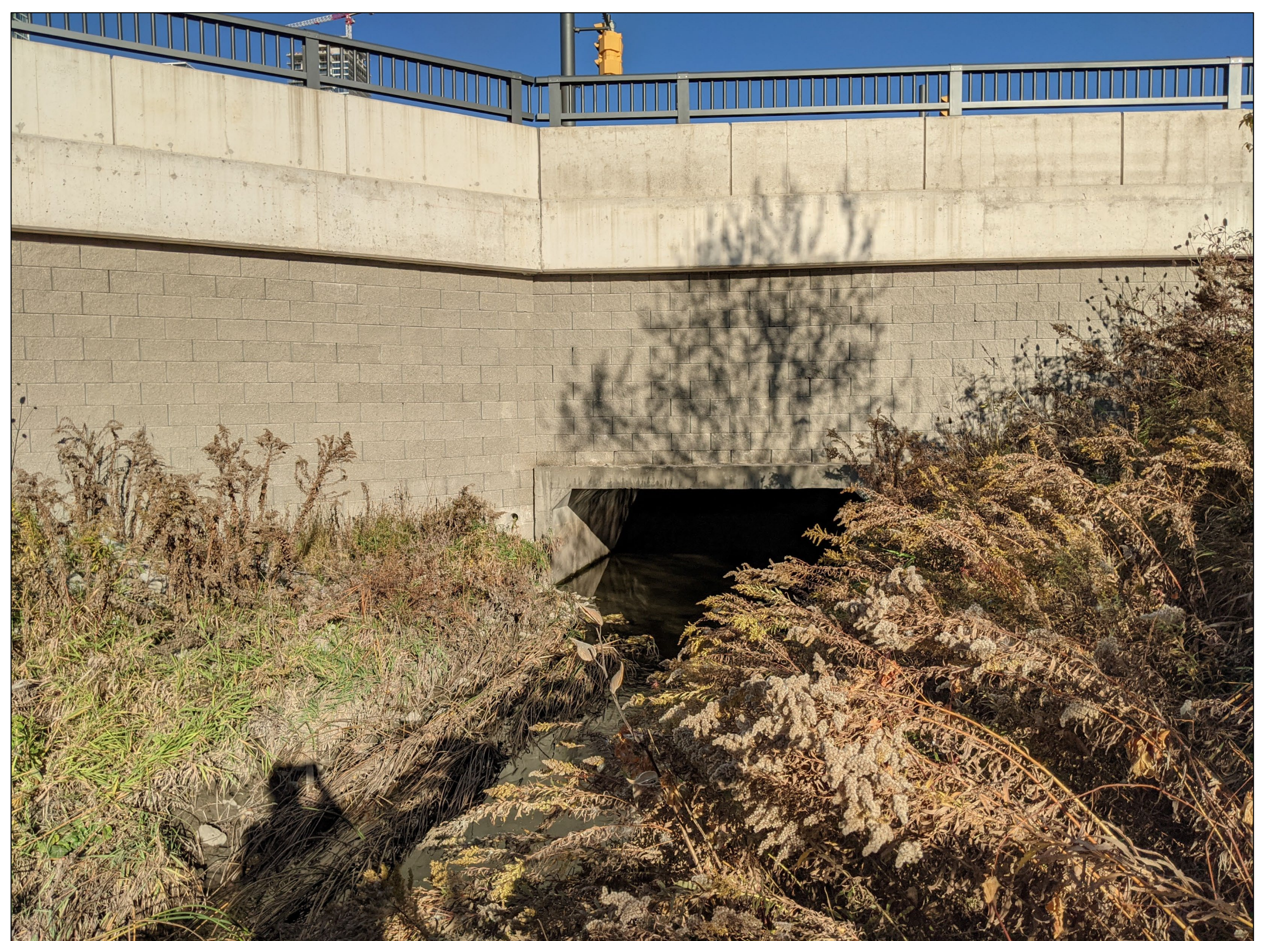
Facing north looking at existing Highway 7 culvert flowing south
