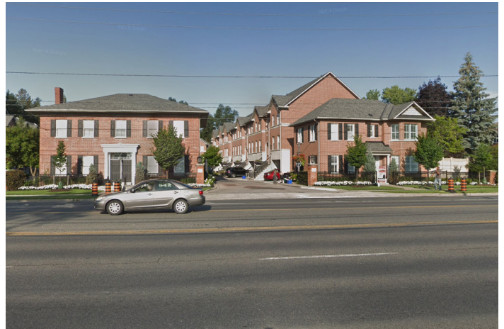
Figure 10. North Area - residential homes addressing Yonge Street
