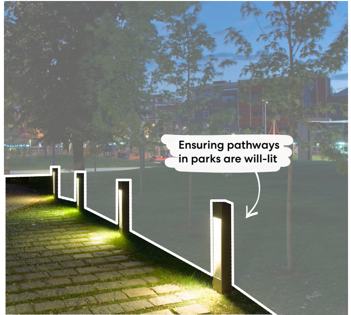
Figure 66. Topa Urban Lighting for lighting pathways in parks source: Designboom
