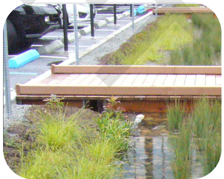
Figure 67. Rain gardens should contain hardy plantings that can withstand drought and flood conditions
