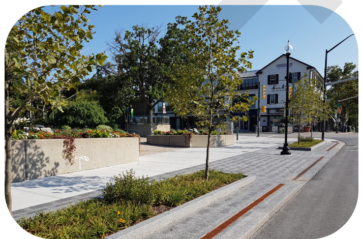
Figure 106. Low-level planting beds ensure more surface water retention and air circulation for street trees.
