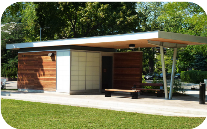
Figure 127. A simple expansion of the roof can provide shade and weather protection to support small amenity areas
