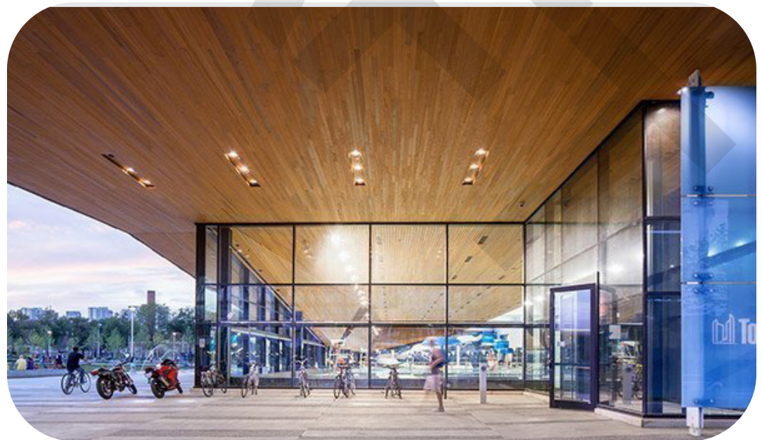
Figure 65. Entrance to a Community Building with significant glazing and bicycle parking to promote active transportation
