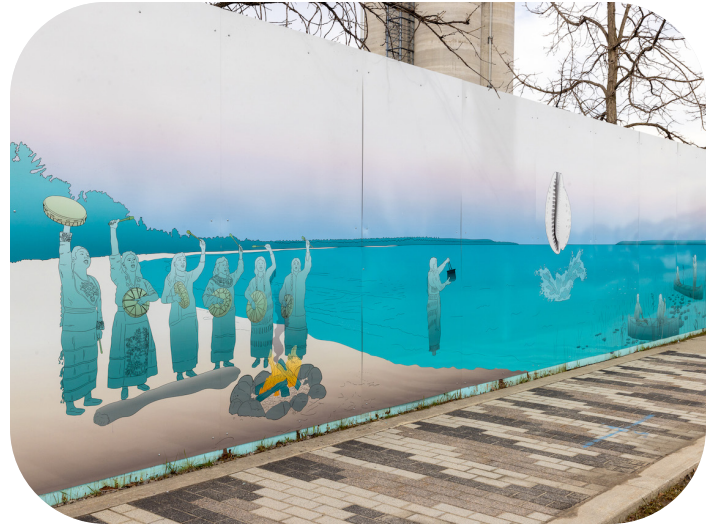
Figure 147. Construction hoarding can provide an opportunity to enliven space and share information through public art and signage.
