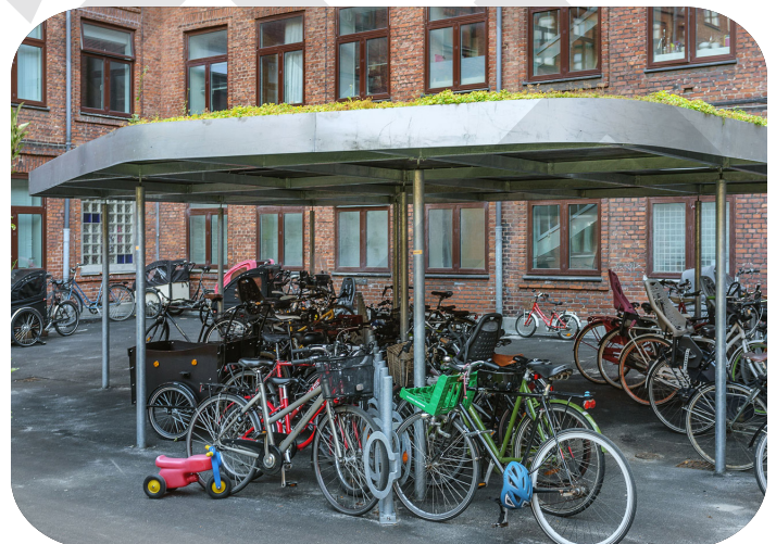
Figure 123. This bicycle shelter incorporates a green roof structure
